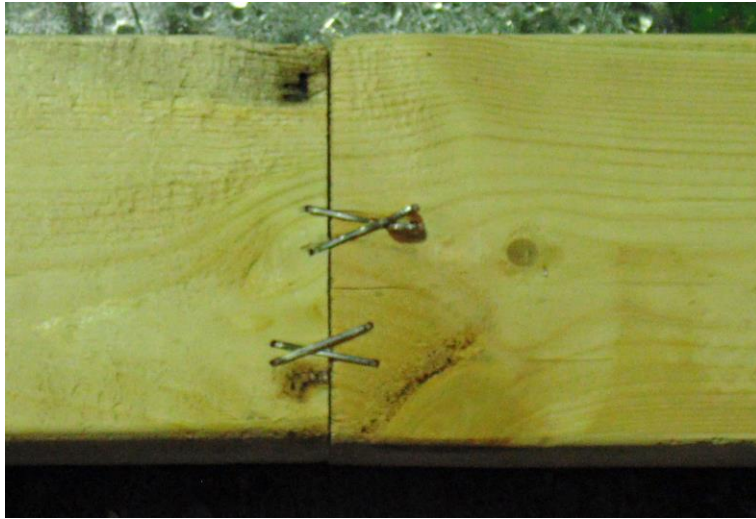
Proper stapling of a joint using a X pattern
