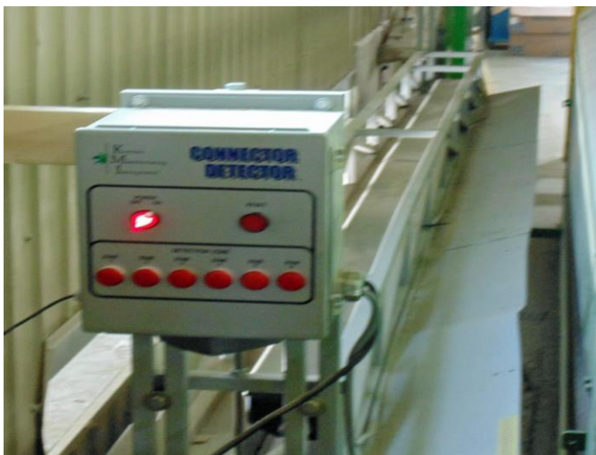
Installed Metal Plate Detector after the finishing roller
