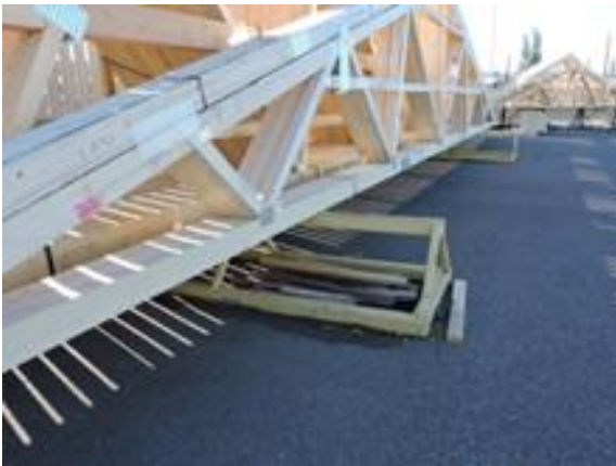
Trusses stacked vertically and horizontally
