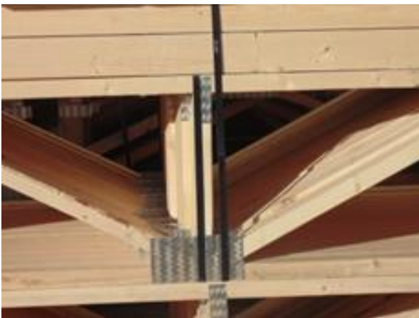
Proper banding at the post
