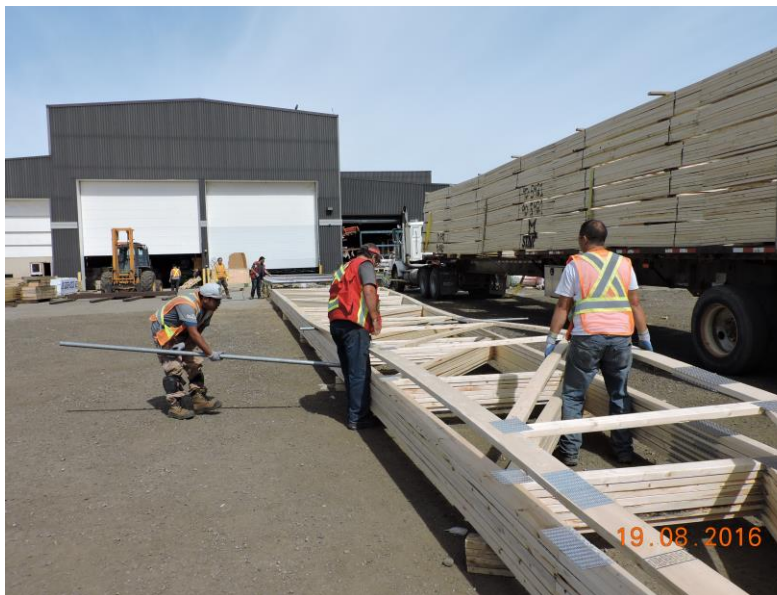
Using pipes as temporary rollers
