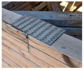
Examples of trusses that have been sitting in a yard and the plates have withdrawn making the teeth ineffective.
