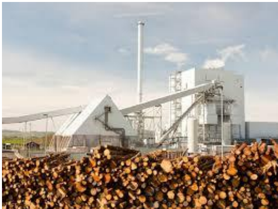
Biomass Power Plant
