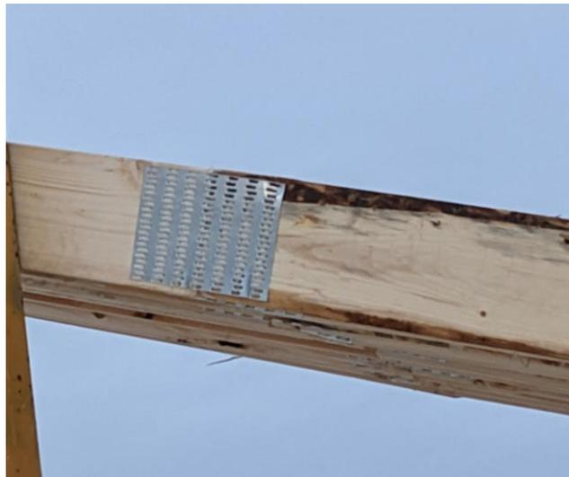
In the case of the picture above there was a defect (wane) reducing the number of effective teeth into the top chord and the plate should have been upsized to take this into account. Because it was a butt cut the web could only be placed in this orientation as the other end had a plumb cut at the overhang.
