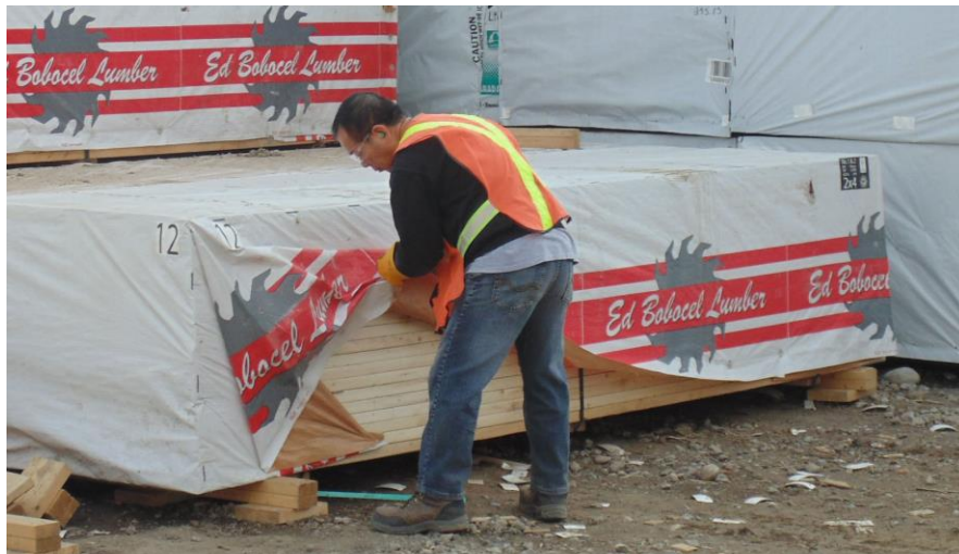
Lumber being unwrapped and on proper dunnage off of the ground.
